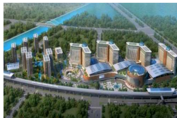
The First Affiliated Hospital of Zhengzhou University —The Largest Hospital in the World
